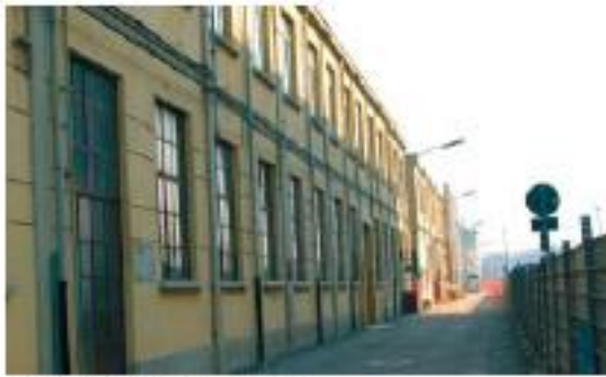
Pirelli building prior to demolition
