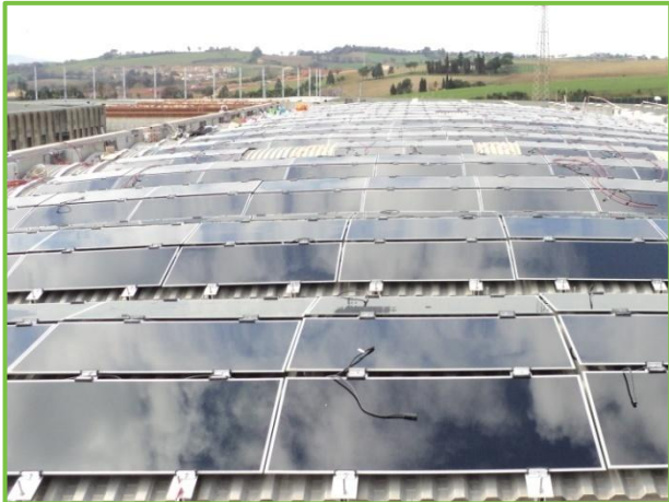
First Solar rooftop installation
